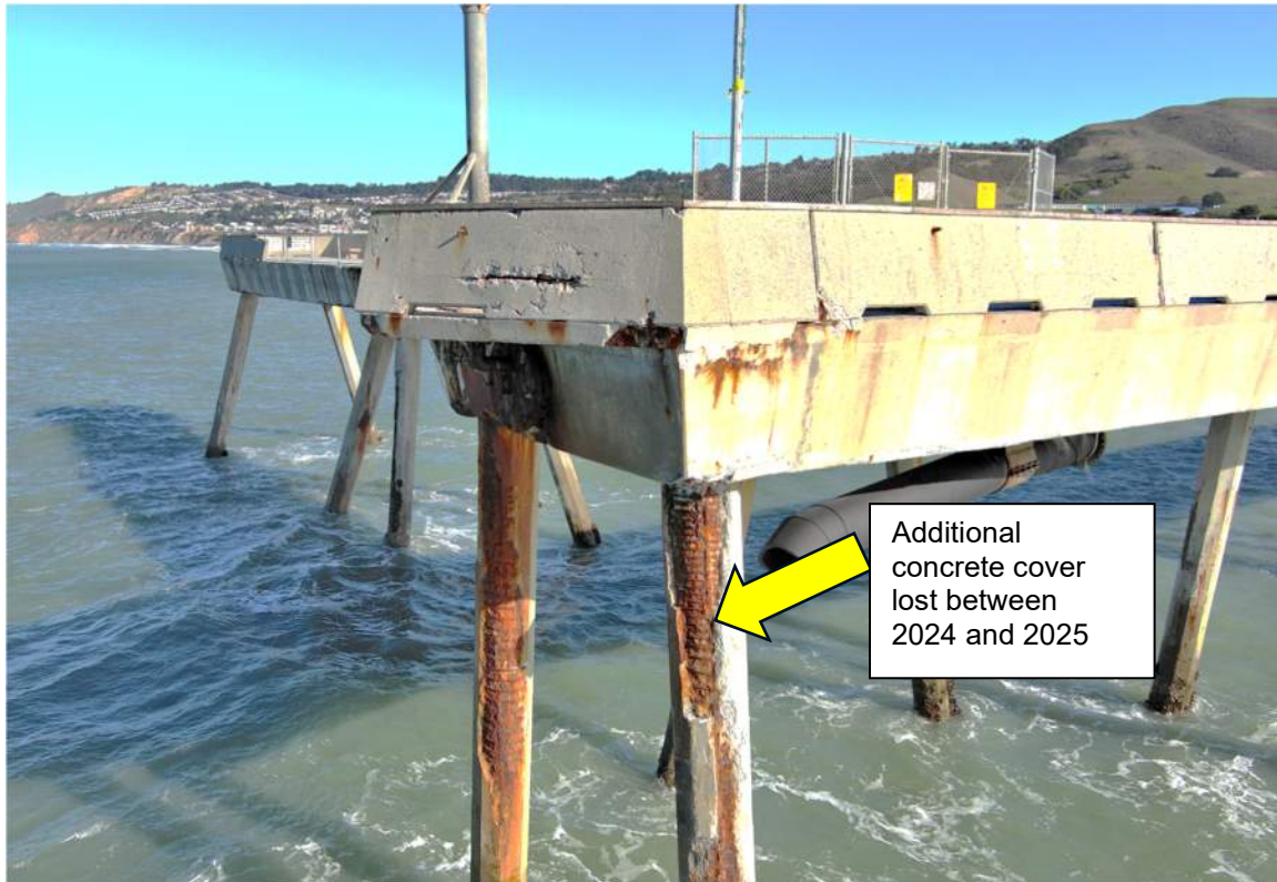
Figure 3.4 Pile and Outfall Pipe at Bent R in January 2025
