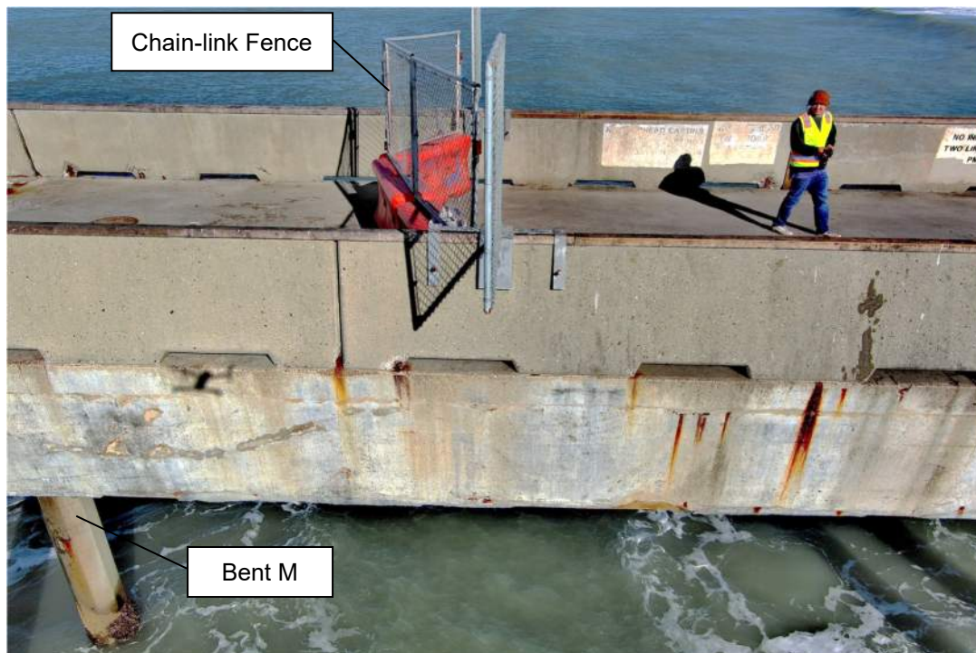
Figure 1.2 Chain-link Fence on Main Pier near Bent M
