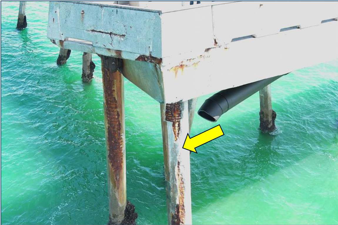
Figure 3.5 Pile and Outfall Pipe at Bent R in April 2024
