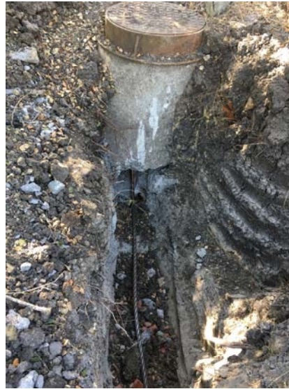
3. Pull wire laid in pipe
