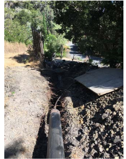
4. New pipe pulled
