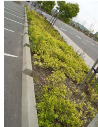
Parking lot drains to planter strip, Millbrae
